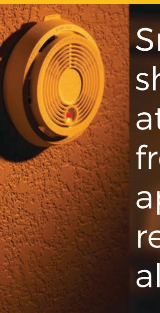
Smoke alarms should be placed at least 10 feet from cooking appliances to reduce false alarms.
